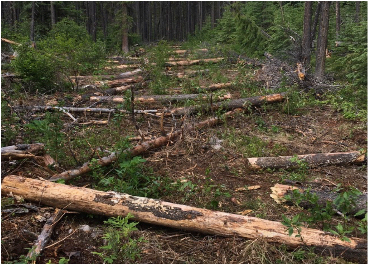
Photo 13: Machine screefing and debris rollback on Line Segment #74.
