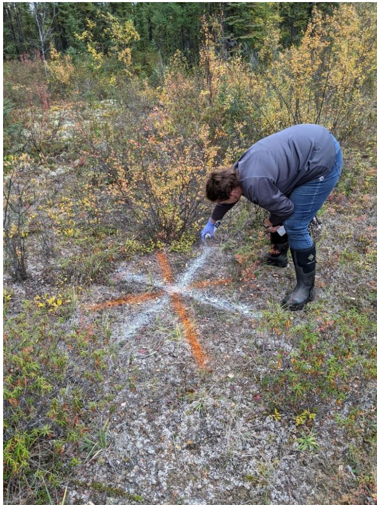
Figure 14. Spray painting a ground control point.
