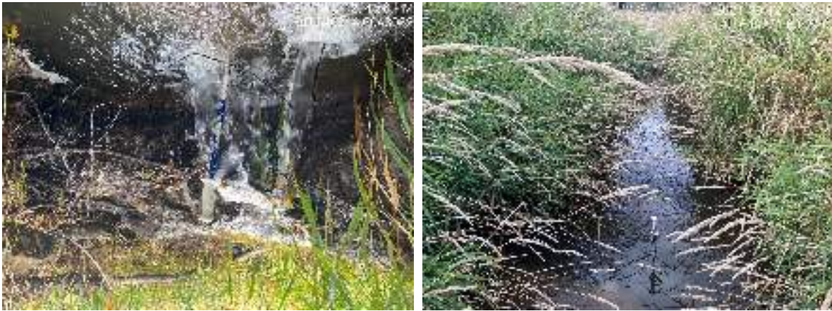
Figure 5.47: Left: Small drop (50cm high) located ~20m upstream of PSCIS crossing 198066. Right: Habitat immediately upstream of PSCIS crossing 198066 that flows through a hay field within an excavated trench for approximately 350m.
